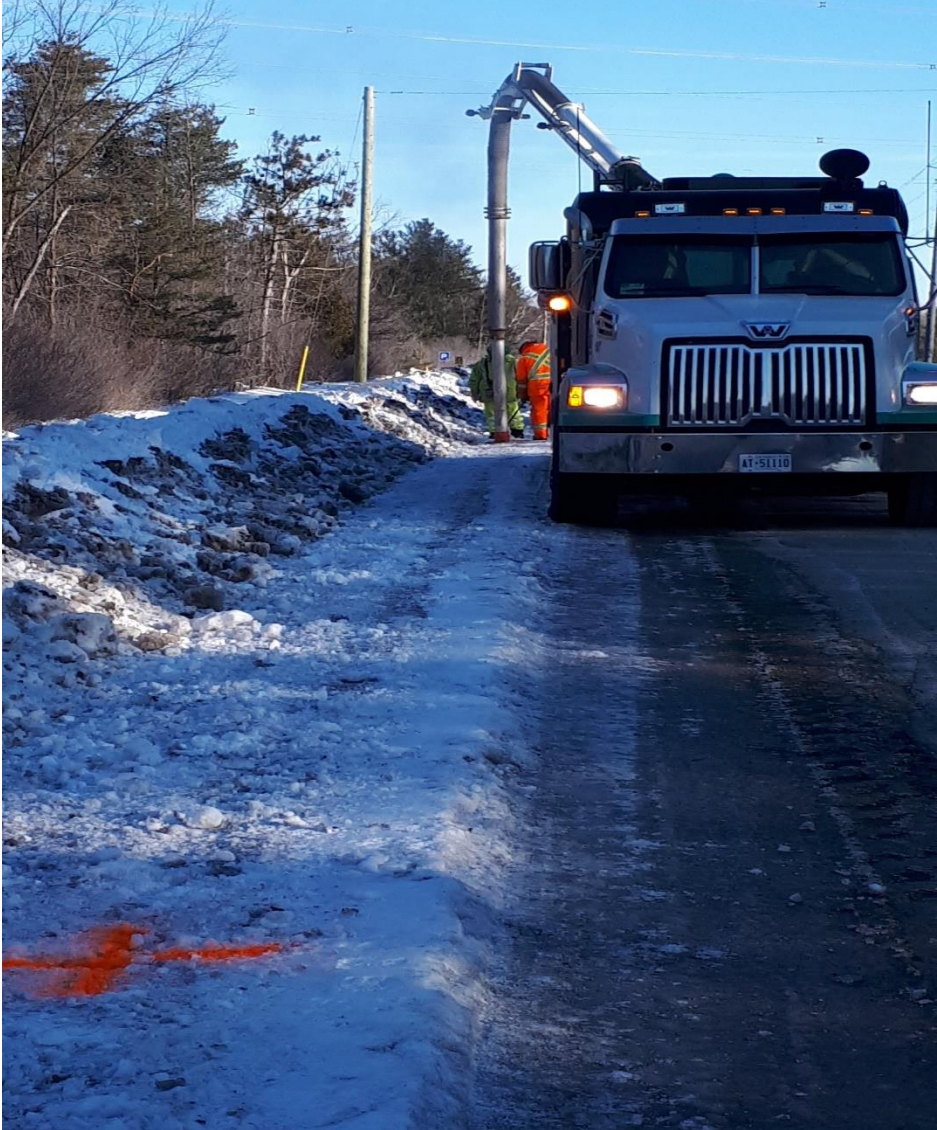
Picture 2: Tests Pits to Locate Main Gas Lines
