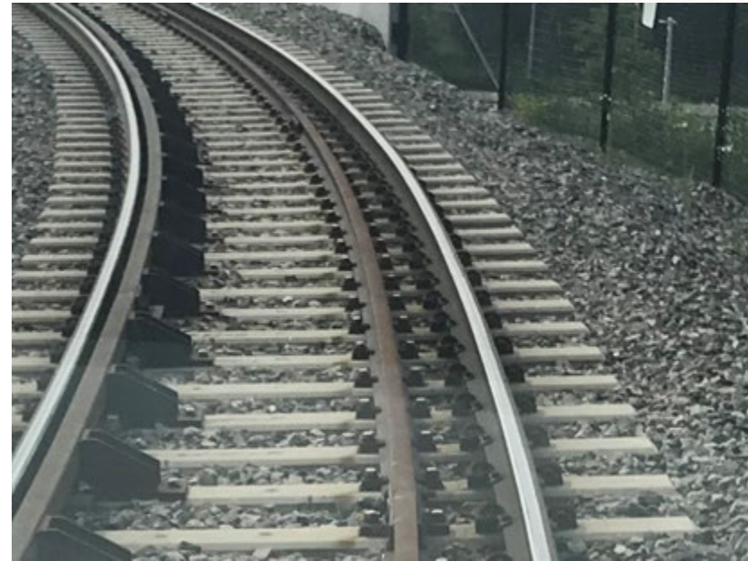
Fig. 1 welded track (above)
