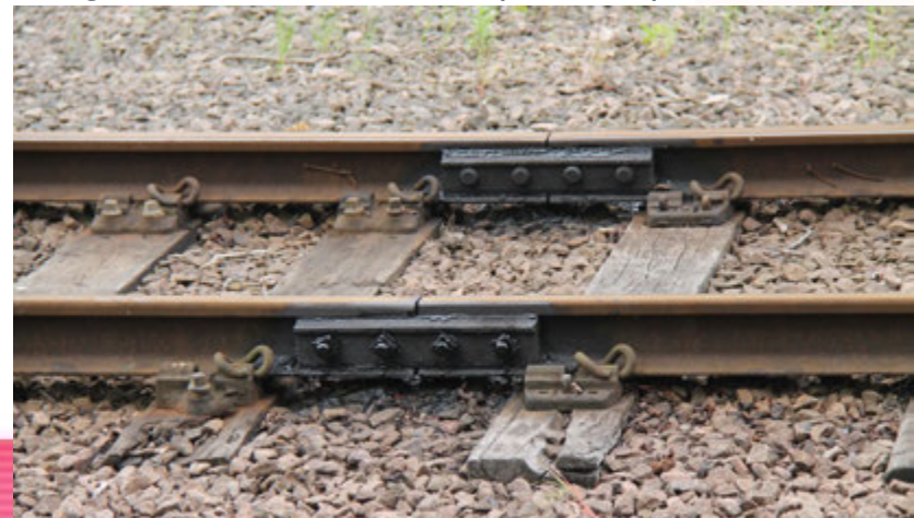
Fig. 2 jointed rail
