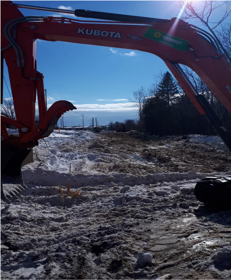
Picture 1: Clearing and Grubbing Adjacent to Old Richmond Road
